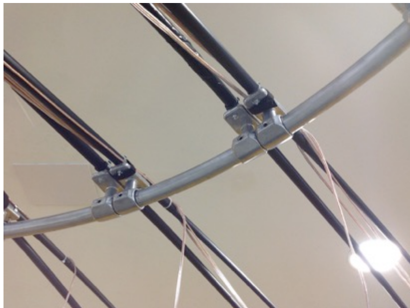
Figure 3; Detail of whips fixed to circle
